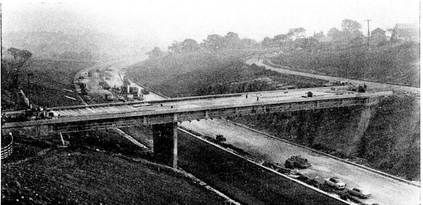
Hill Top Bridge and Cutting under construction - Contract M61/6
